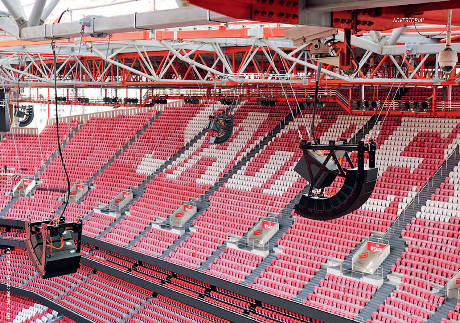
d&b A-Series augmented array and XSL cardioid line array
