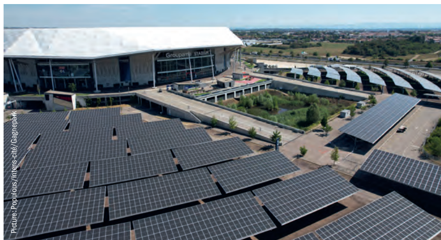
Huge photovoltaic system near the Groupama Stadium.
